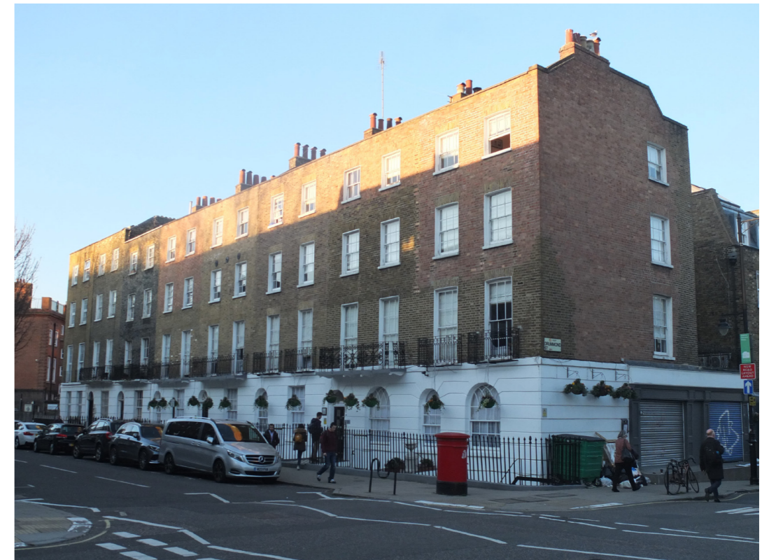
grade II listed (Georgian) Regency terrace
