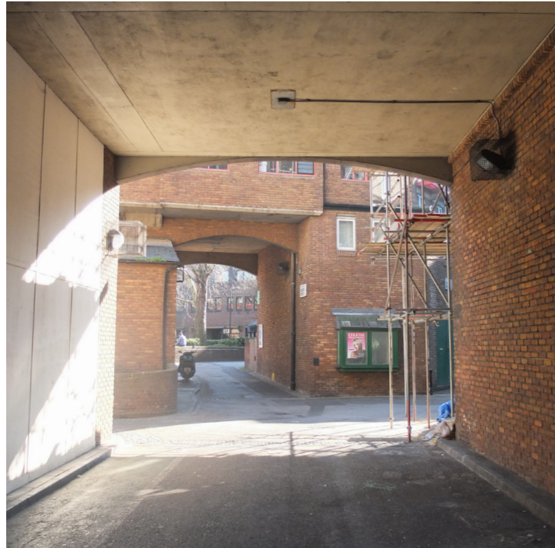
underpass leading from the high street to Tolmers Square
